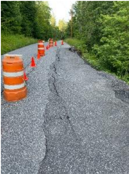
Fluvial erosion has caused a slump and damage to pavement on Bosley Hill Road in Readsboro. Photo courtesy of Omar Smith.
