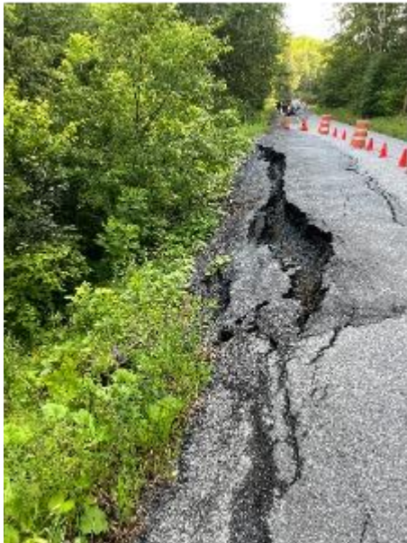
Fluvial erosion damage has caused a slump and damage to pavement on Bosley Hill Road in Readsboro. Photo courtesy of Omar Smith.
